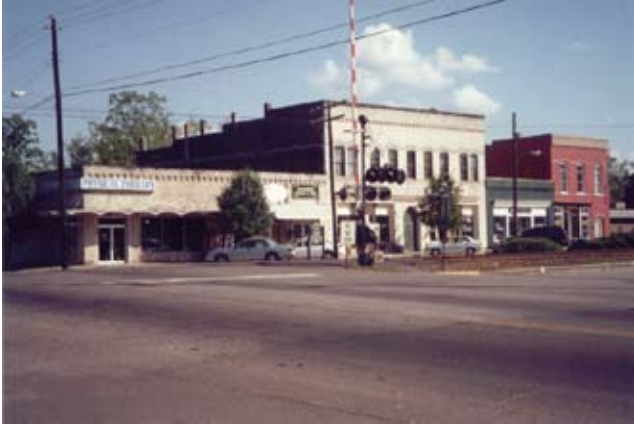
This is a view of the downtown area prior to construction
